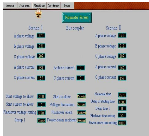
FIGURE 2 Monitoring menu of the power network status
